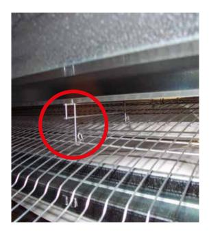
At the same time, this "hookup" system creates a rigid joint to the structure of the battery and therefore it allows to have great stability even if submitted to transversal stress.
